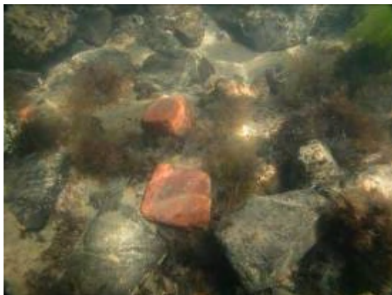
Rock and Bricks at Base of Revetment
